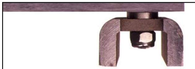
Fig. 17: Supported by 316 stainless steel channels, the FRP holder for each ceramic cover strip is retained by removable studs. The stud shoulder takes loading strains off the holder to prevent cracking or splitting.
