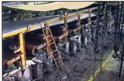
The No. 3 paper machine wet end at Los Reyes consisted of nine conventional counterflow vats and one dry vat which formed board from 55 to 110 pounds per 1000 square feet (#/msf). Production speeds range from 250 to 450 feet per minute
